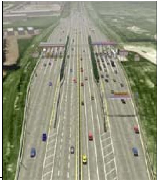
Figure 2: Ariel View of Open Lanes on Illinois Toll Highway (3)
