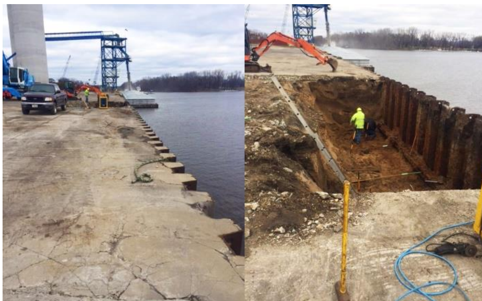
Work underway to repair dock wall failure at F.J. Robers in La Crosse.
